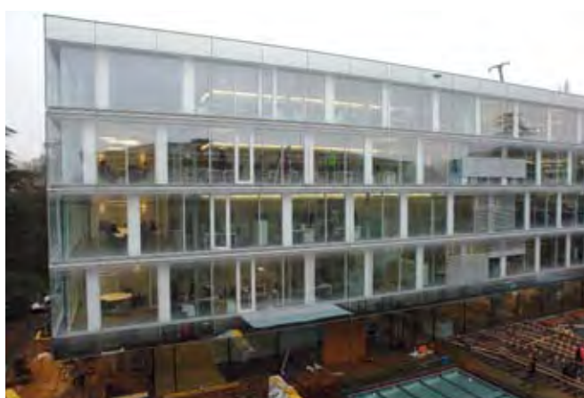
In 2012, work on the annex at the WTO's Geneva headquarters was completed, putting all staff under the same roof for the first time.
