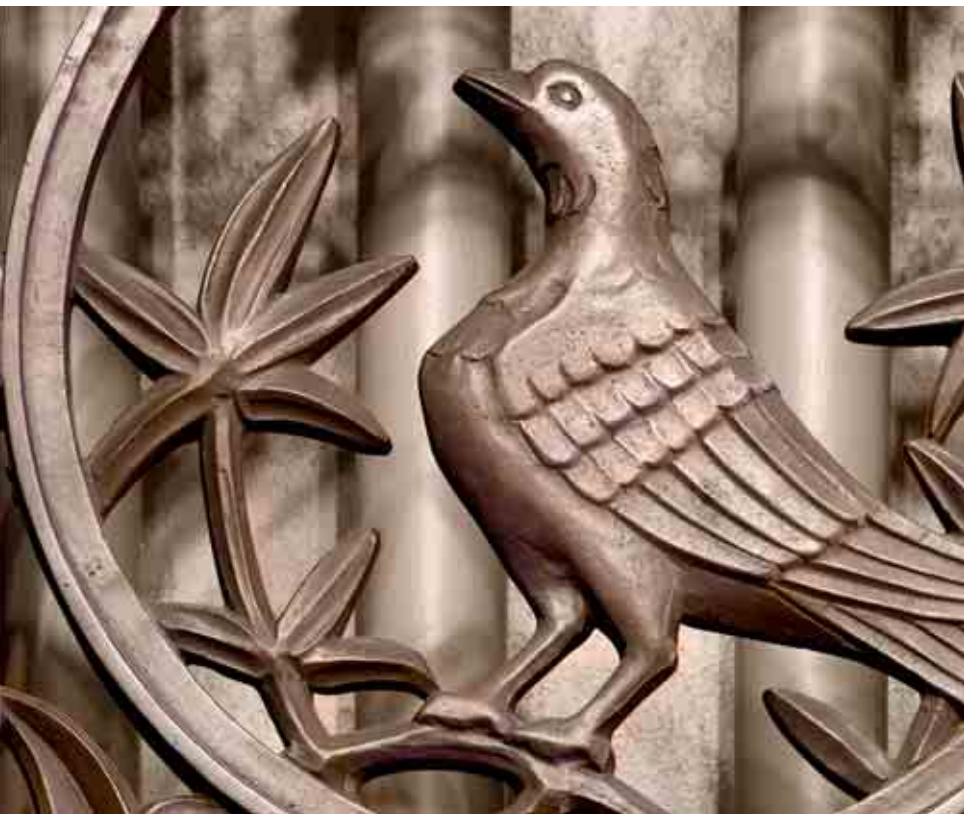
Ironwork, in main entrance (Uberti, 1926)
