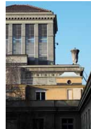
➤ The northern tower in the main entrance hall
