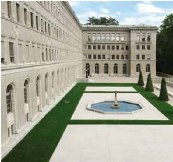
➤ A north-facing view of the lakeside terrace (© WTO/Koen Van Beversluys)
