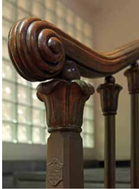
↗ Base of ground floor stairway bannister, south-east corner of the original building (locksmith Edmond Hess, 1926)
