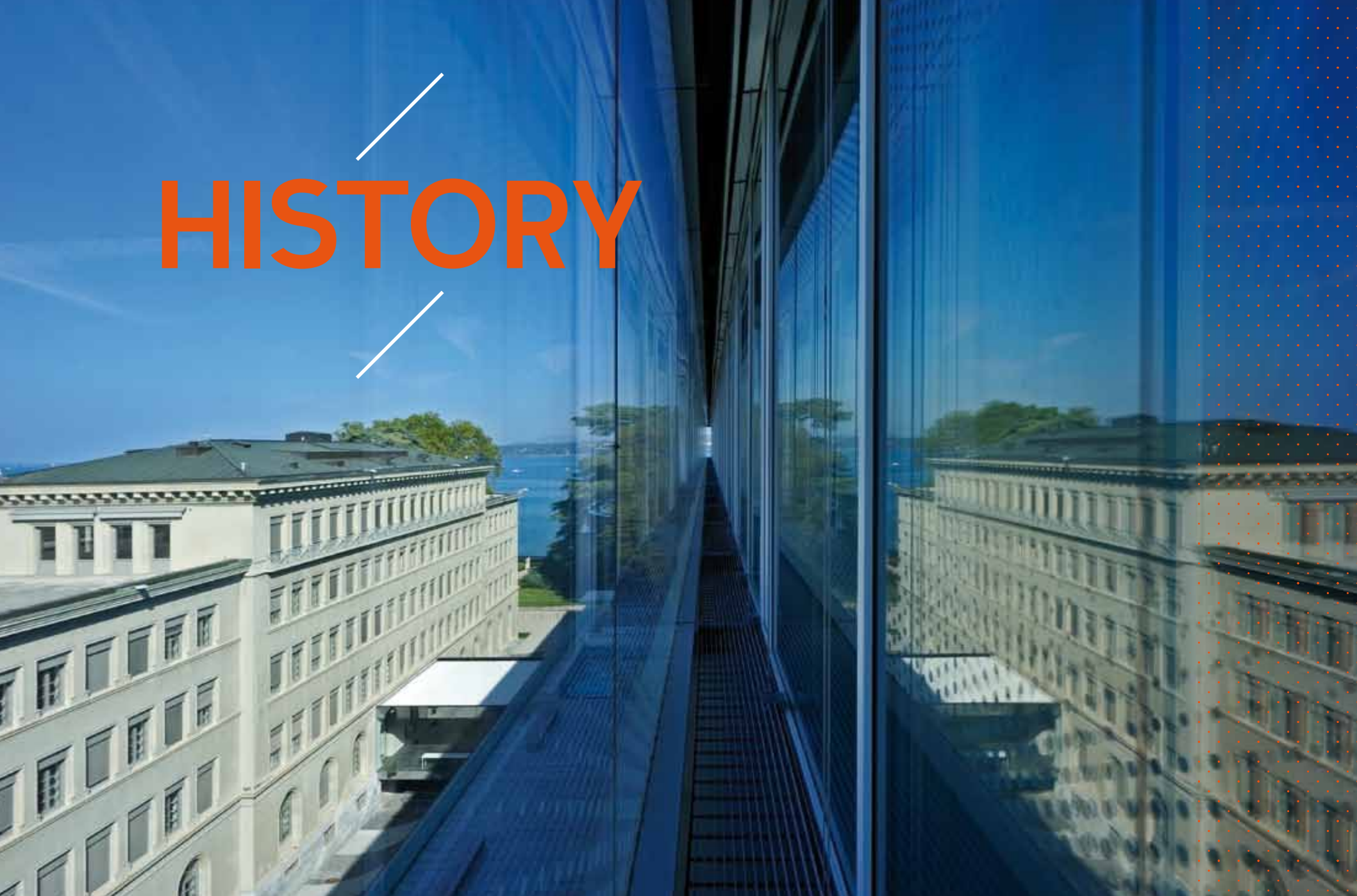
The view between window panes in the South Building
